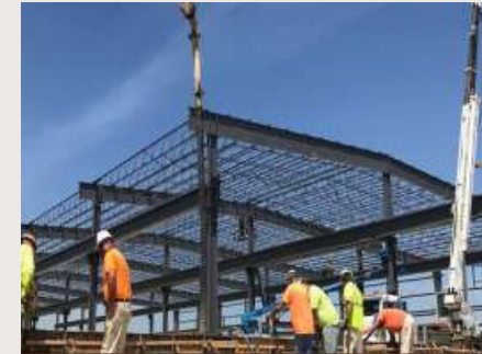
INDUSTRIAL CONSTRUCTION PROJECTS: 9
